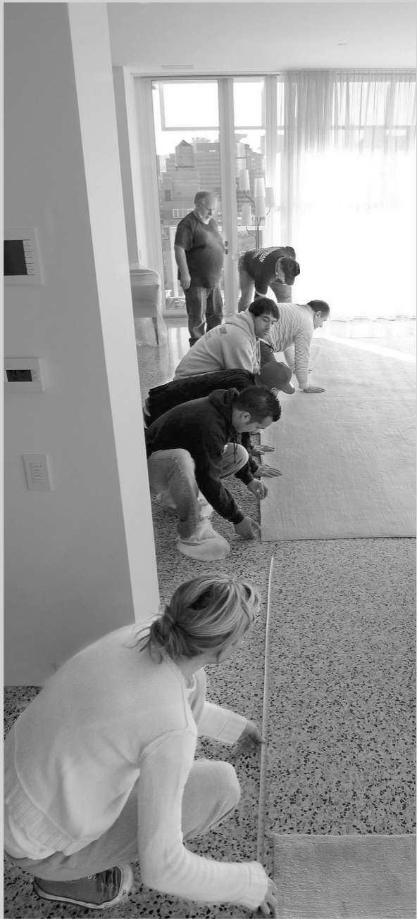
Alexis and crew making sure the carpet is aligned properly.
