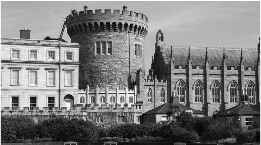
The Record Tower (center) is the sole surviving tower of the medieval Dublin Castle dating from ca. 1228. To its right is the Chapel Royal.
